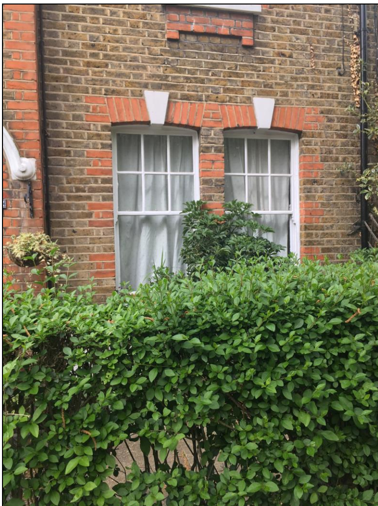
Figure 16: Traditional timber sash windows
