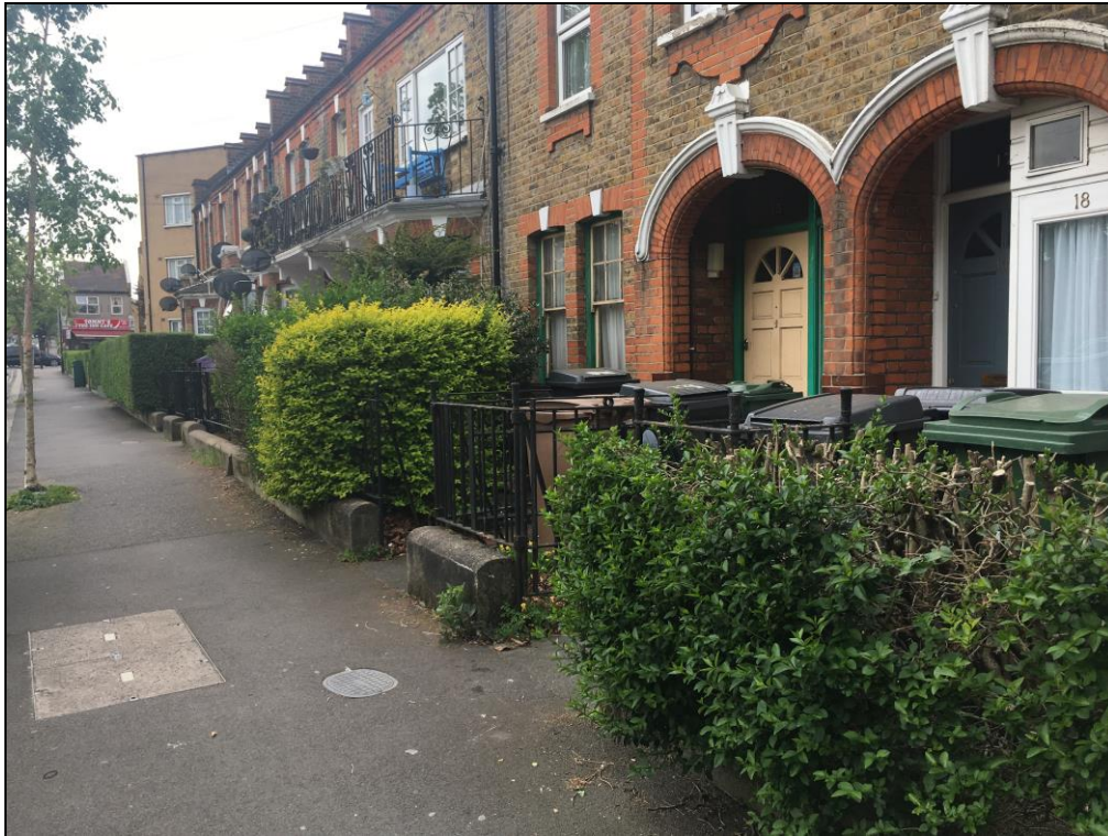
Figure 20: Wheelie bins partially screened by hedge planting
